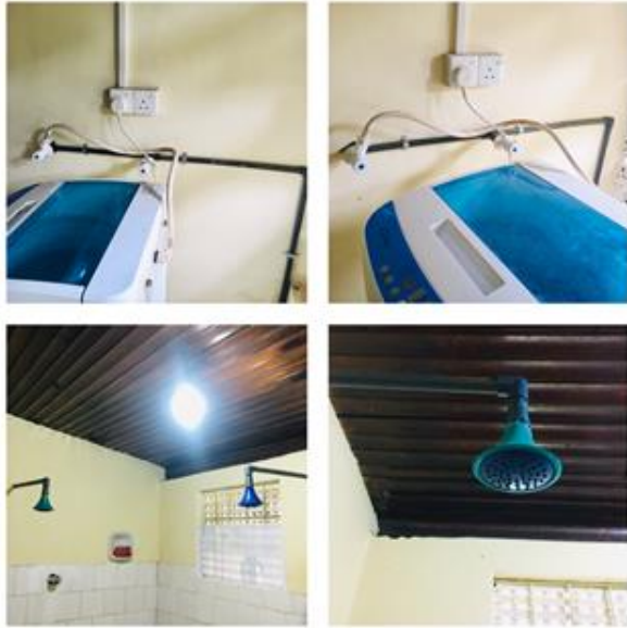
Picture – Upgraded Showers, Tap lines
