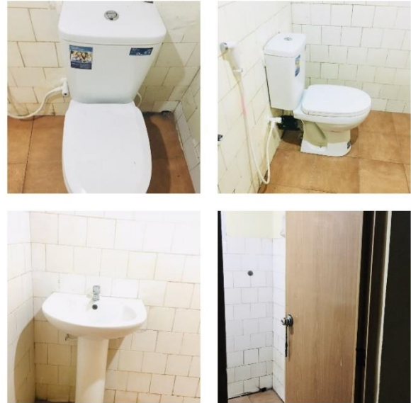
Picture – New doors, sinks and toilets
