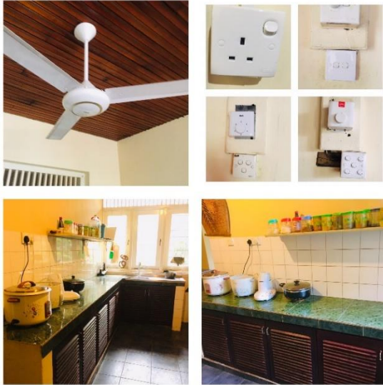
Picture – New pantry cupboards, fan, repaired plug points,
