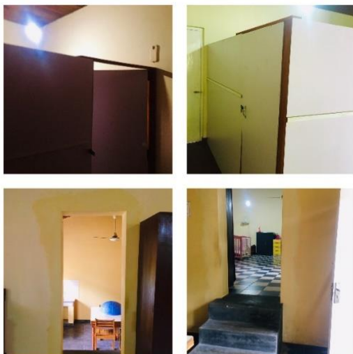
Picture – partitioned rooms, staircase and doorway
